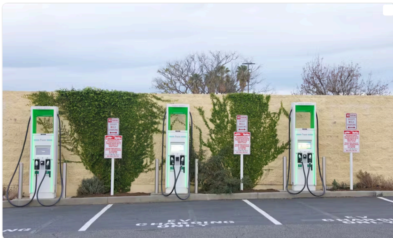
FIG. 1. Electric vehicle charging stations will add DC power demands to buildings.
